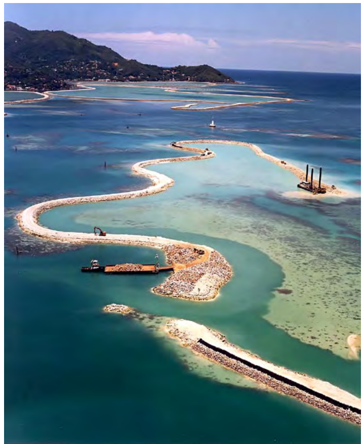
Dredging and reclamation near coral reefs off Mahe, Seychelles, 2003. Jan de Null Group.
